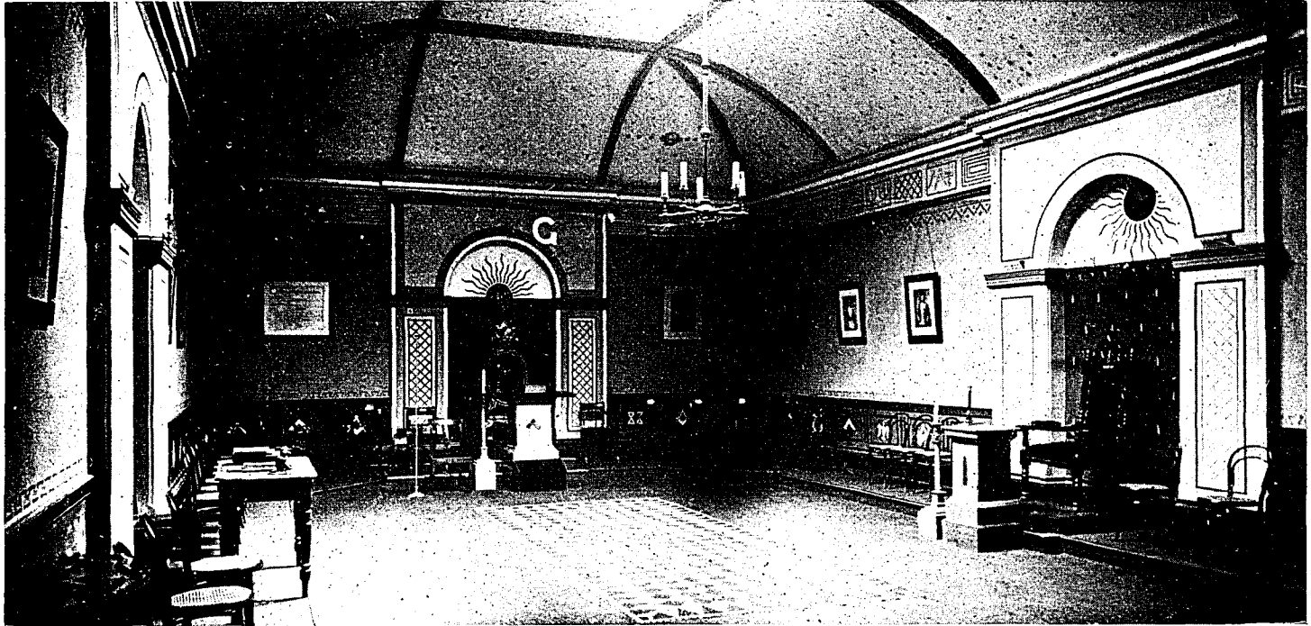
MASONIC HALL, ILFRACOMBE (LOOKING EAST).
